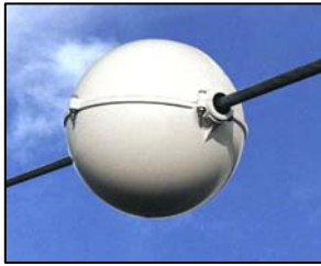
BALISAGE DIURNE < 132 kV
